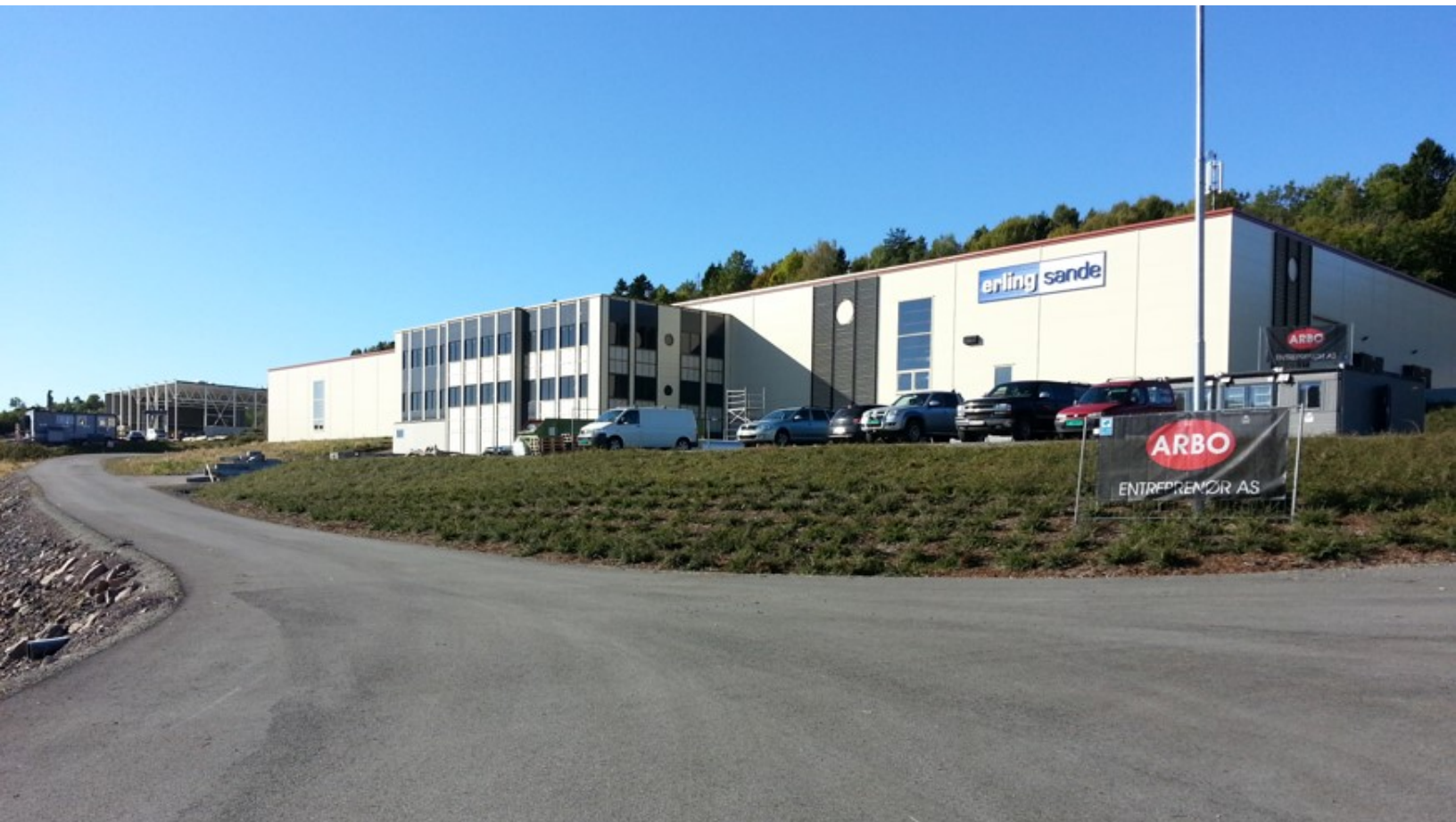
Erling Sande AS headquarters - Drammen, Norway
